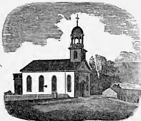
St. Peter's Church, erected in 1790.
